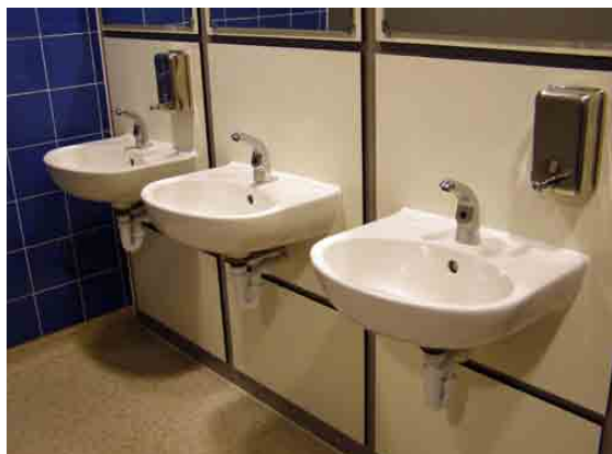
Independent panelling systems protect pipework and simplify surface cleaning
