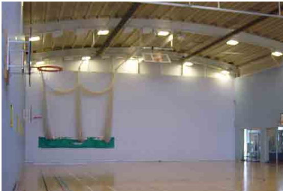
Light fittings suspended from main beams located between the badminton courts. Additional lighting for cricket nets.
