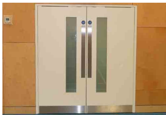
Standard proprietary flush door with a flush viewing panel, opening outwards away from the sports hall
